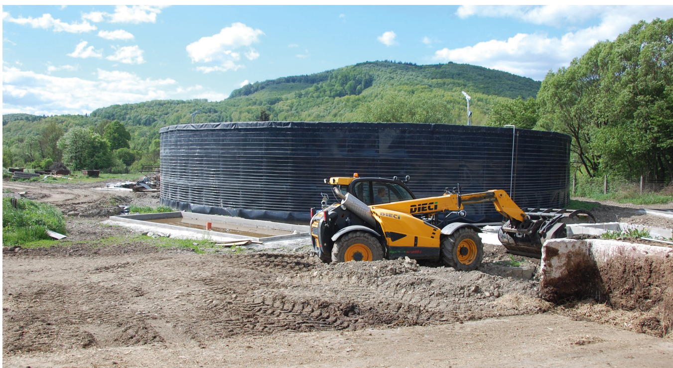
Large-capacity manure tank with manure separator under construction.
